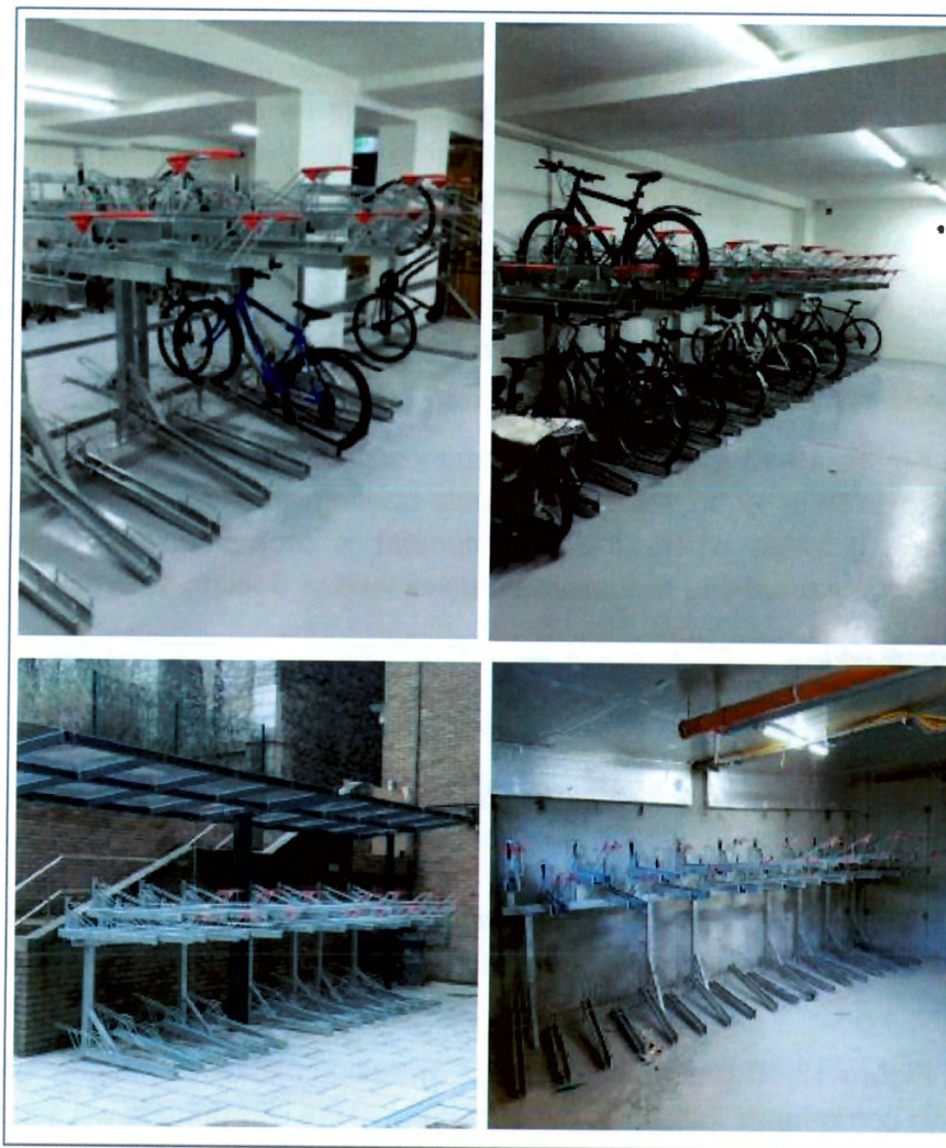
Figure 13-14: Double Stacked Cycle Parking Layout
